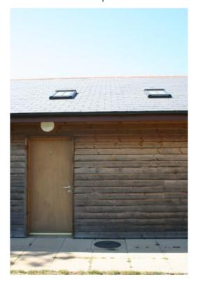
The lower boards are particularly vulnerable not only to direct rain exposure but also to the rebounding of water from the hard paving which the boarding nearly touches.
